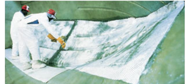
*Skilled craftsmen apply hand laid fiberglass with precisely the right thickness and resin ratios. Top quality components assembled with skill result in quality, reliability and performance over the long haul.*
